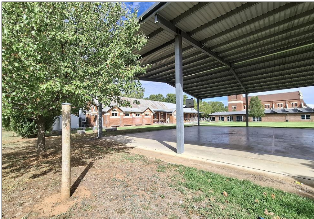
Figure 7 – Site Photo – View looking from the front setback to the west, with the existing COLA in front and existing buildings behind including De La Salle Brothers' School building and Church
