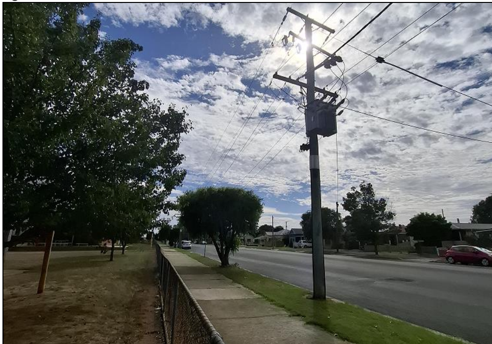
Figure 9 – Site Photo – View looking along the verge of the subject portion of the site with existing overhead electricity lines and poles, footpath and street tree, Sutton Street on the right and trees within the front setback on the left
