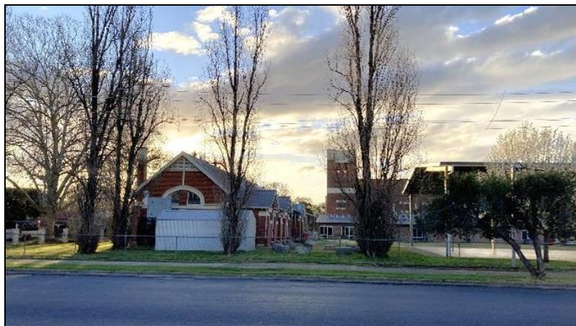
Figure 14 – Site Photo – View looking from the front setback, with the existing COLA on the right and existing De La Salle Brothers’ School building on the left and Church visible behind
